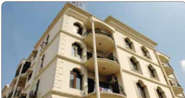
Vintage Apartment | 📍 Butler Road, Lucknow
