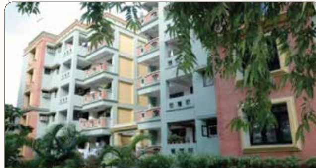
Pashupati Apartment | 📍 Way Road, Lucknow
